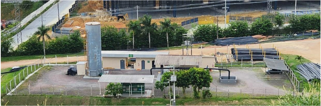
Figure 2 – Gas Regulation Station.
